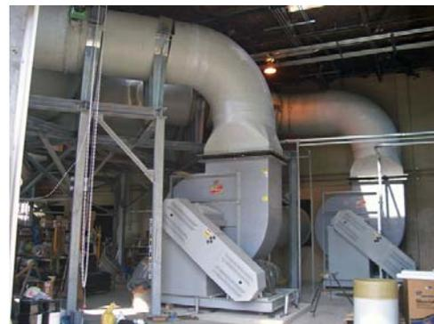
Composite ducting moves air toward the stacks.
